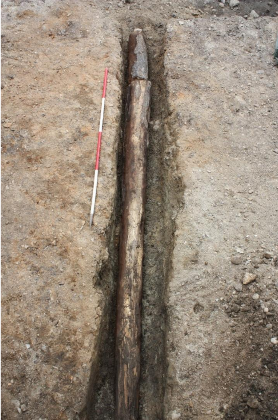
Fig. 287. Exposed water pipe (ST90718), facing north. Photo: Museum of Copenhagen.
