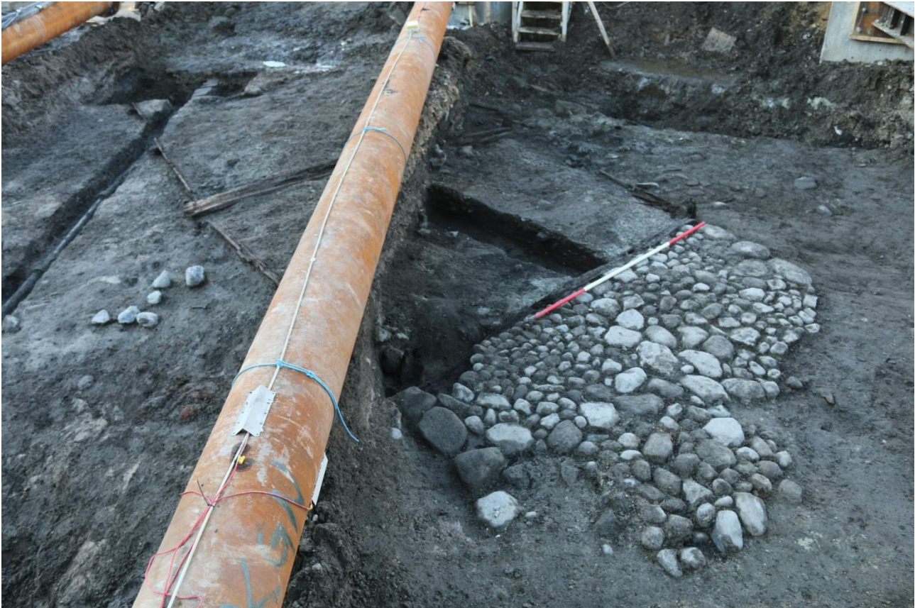
Fig. 316. Overview timber structure with drainage, bedding layers and cobble surface (SS314711), facing SE. Photo: Museum of Copenhagen.
