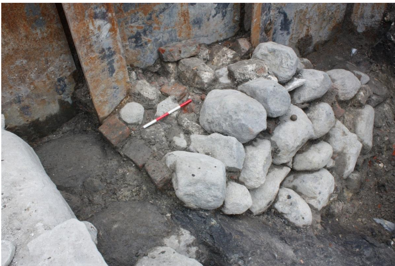
Fig 199. Bricks and stones (SD85806) placed in position behind larger stones and against the city wall foundations, facing NE. Photo: Museum of Copenhagen.
