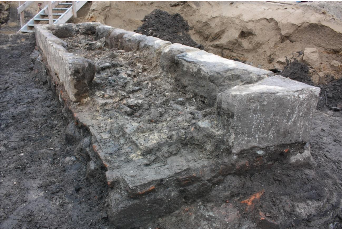
Fig. 233. Bridge pillar No. 2. Part of facing stone wall with ashlar stones SS304186 and rubble infill SS304582, facing north. Photo: Museum of Copenhagen.
