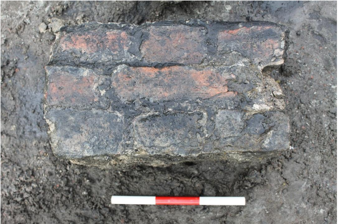
Fig. 225. Building material from the former moat. Masonry (Dutch or English cross bond) from demolished bridge structure, from above. Photo: Museum of Copenhagen.
