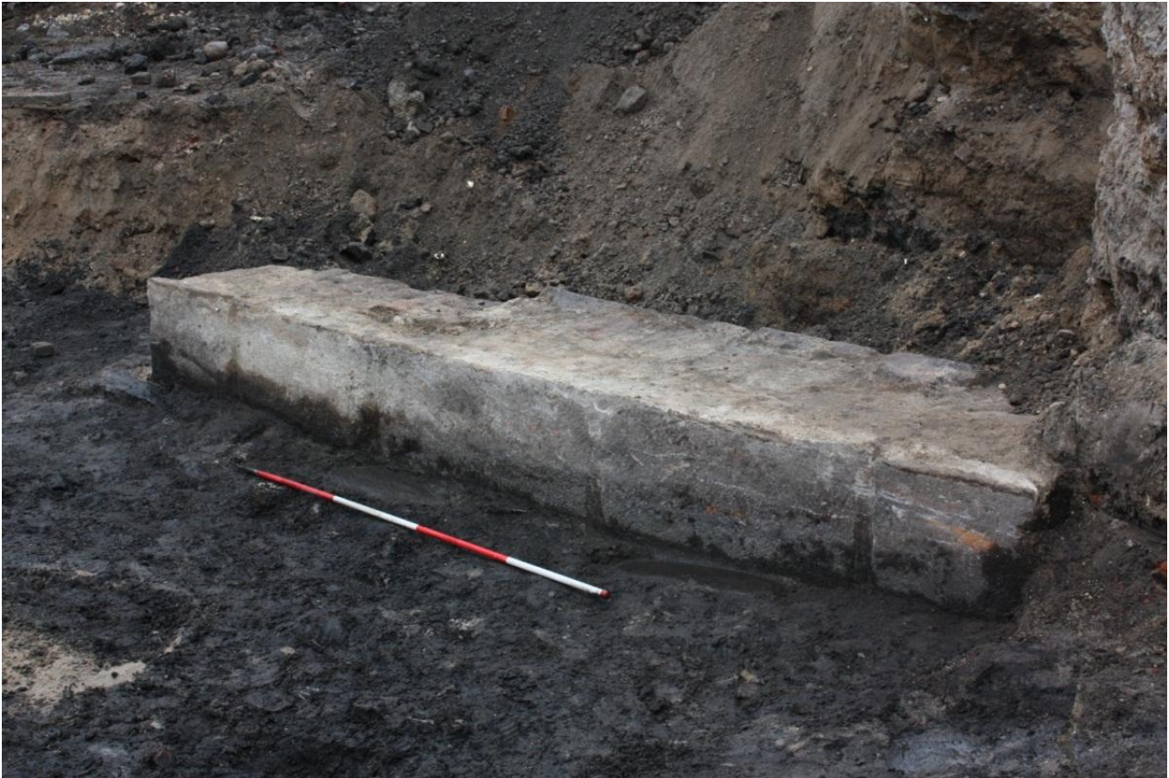
Fig. 230. Continued investigations. Exposed bridge pillar No. 1 (2014) with ashlar stones SS304586 and cemented core of yellow-white mortar, facing SW. NW part not fully exposed due to Station Box limit. Photo: Museum of Copenhagen.
