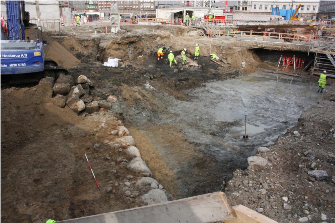
Fig. 216. Investigating the 17 th century fortification step by step. Part of the exposed curtain, facing north. In the middle – staff working on one of the bridge pillars. To the right – the excavated 17 th century moat. Photo: Museum of Copenhagen.
