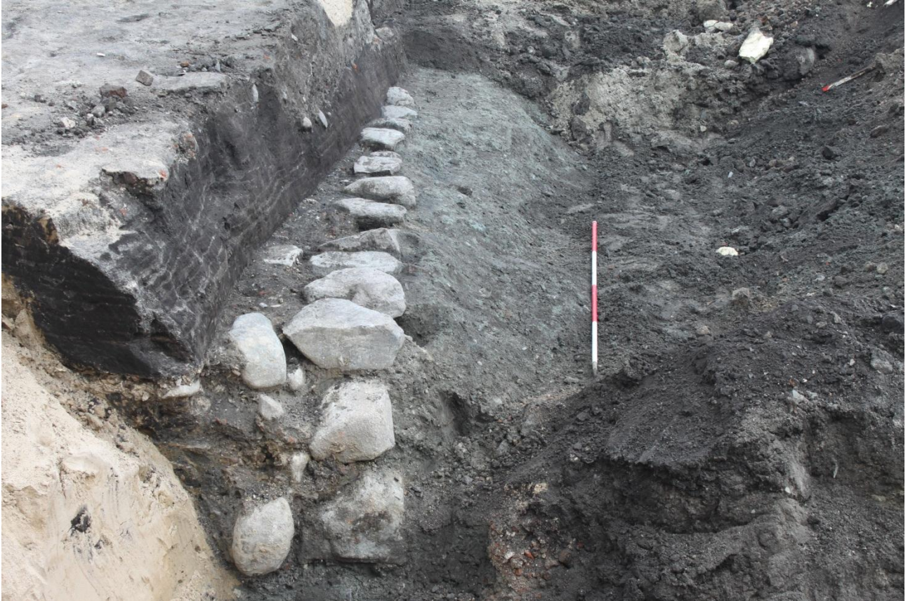
Fig. 207. Southern part of foundation stones SS177220 in the bastion and sealing clay layer SD176814, investigated in 2012, facing NE. Above are multiple layers of peat used as building material in the fortification. Photo: Museum of Copenhagen.
