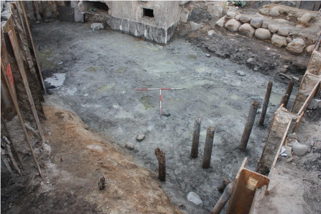
Fig. 144. Excavated 16 th century moat, facing SW. The timber belongs to a later bridge structure. Photo: Museum of Copenhagen.
