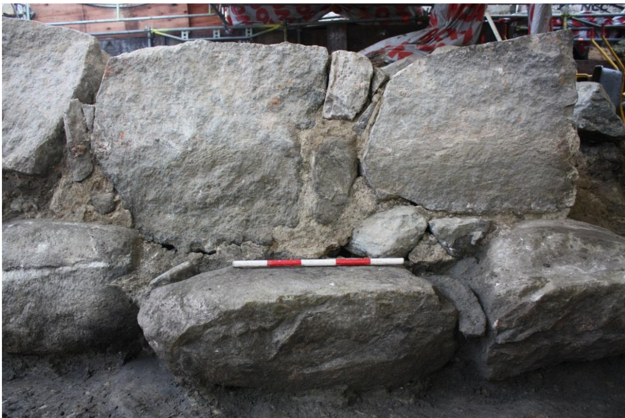
Fig. 130. Extended entrance and rebuilding work in the 1500s? Foundation stones (SS43532) and (SS45115), facing south. Photo: Museum of Copenhagen.
