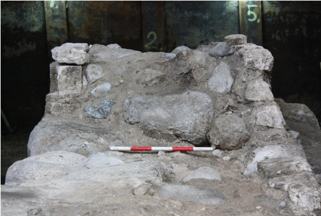
Fig. 106. Cut through the NW gateway showing the two faces of ashlar stones and core consisting of smaller and bigger stones with mortar, facing west. Photo: Museum of Copenhagen.
