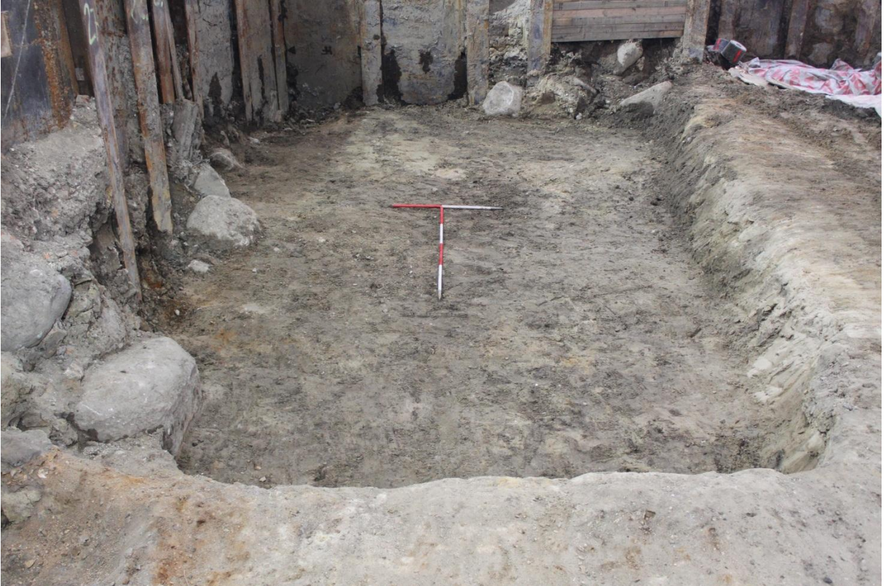
Fig. 99. Post-excavation. Northern construction cut of the gate building without foundation stones, facing east. Photo: Museum of Copenhagen.
