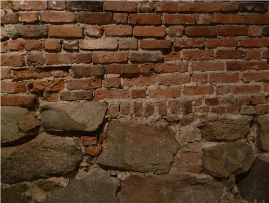
Fig. 97. Example of a Late medieval brick wall. Stockholm's city wall dating from c. 1530 AD. Photo: Morten Steineke.
