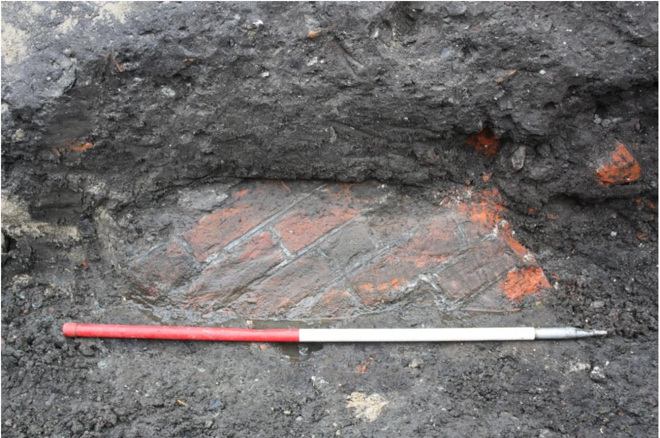
Fig. 86. Monk bond. Part of brick wall (SS24827), facing west. Photo: Museum of Copenhagen.
