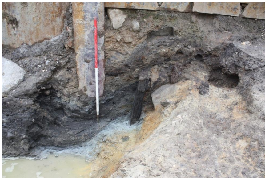
Fig. 70. Interpreted construction cut (SC93401) of the oldest 13 th century moat seen in section, facing south. The bulwark (SG-540) was probably rammed into the base of the cut after the moat was dug, whereupon moat deposits silted up around the timbers as indicated in the section. Photo: Museum of Copenhagen.
