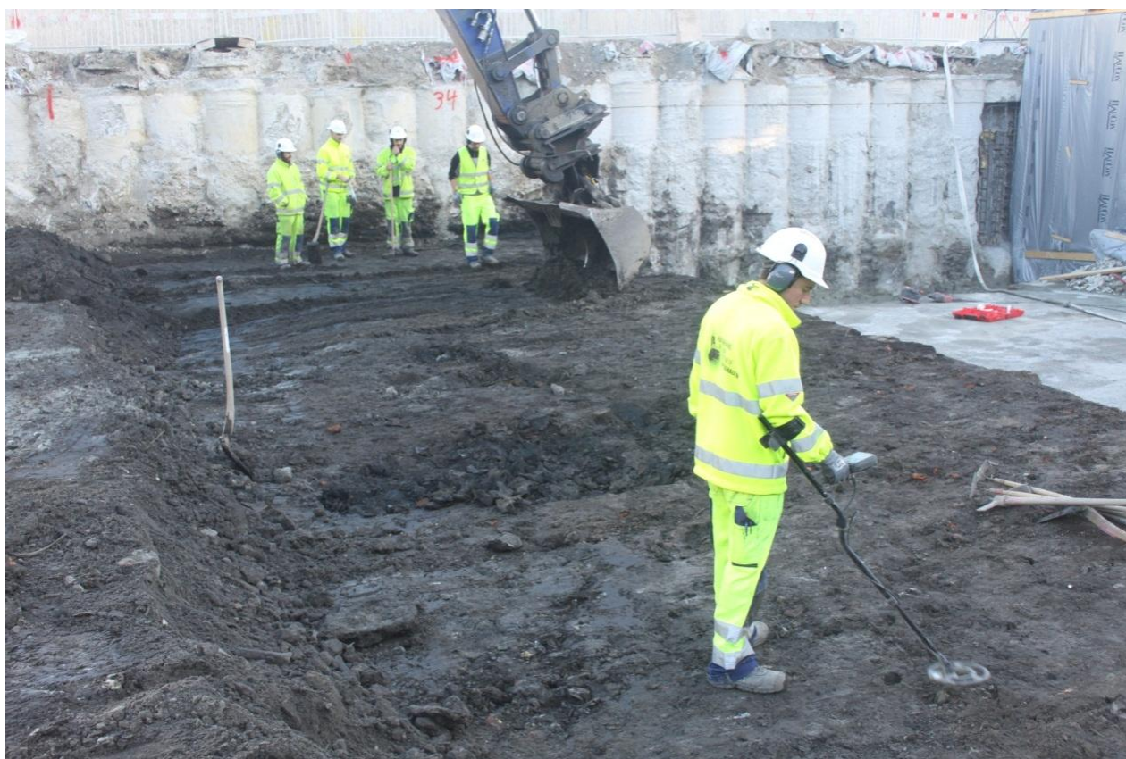
Fig. 17. Machining and metal detecting. Removing larger deposits in the 17 th century moat. Photo: Museum of Copenhagen.
