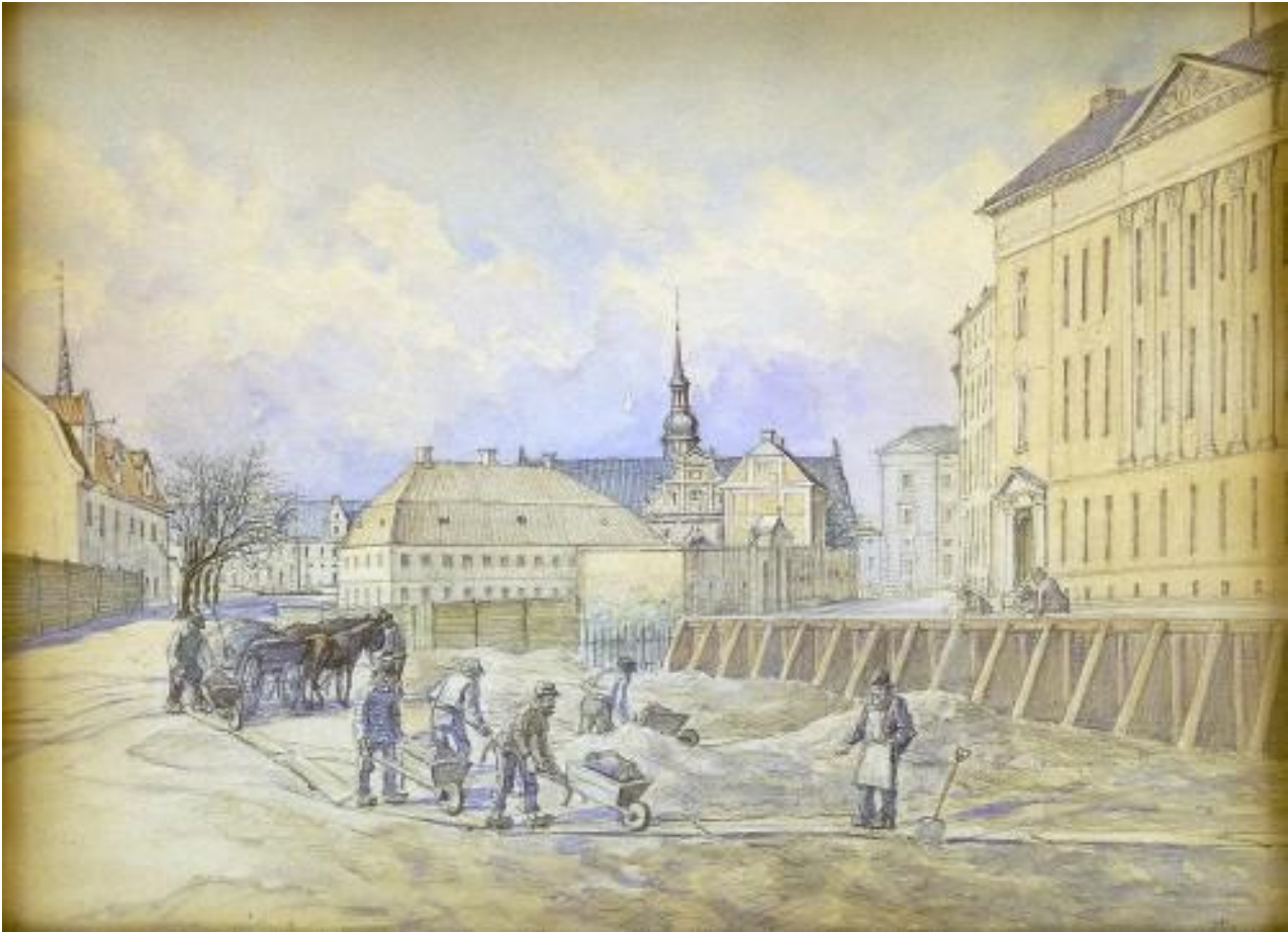
Fig. 344. Removing the last traces of Østervold. Backfilling of Holmens Kanal outside current Danske Bank in 1864 facing Holmens Kirke to the west. Photo: Museum of Copenhagen.
