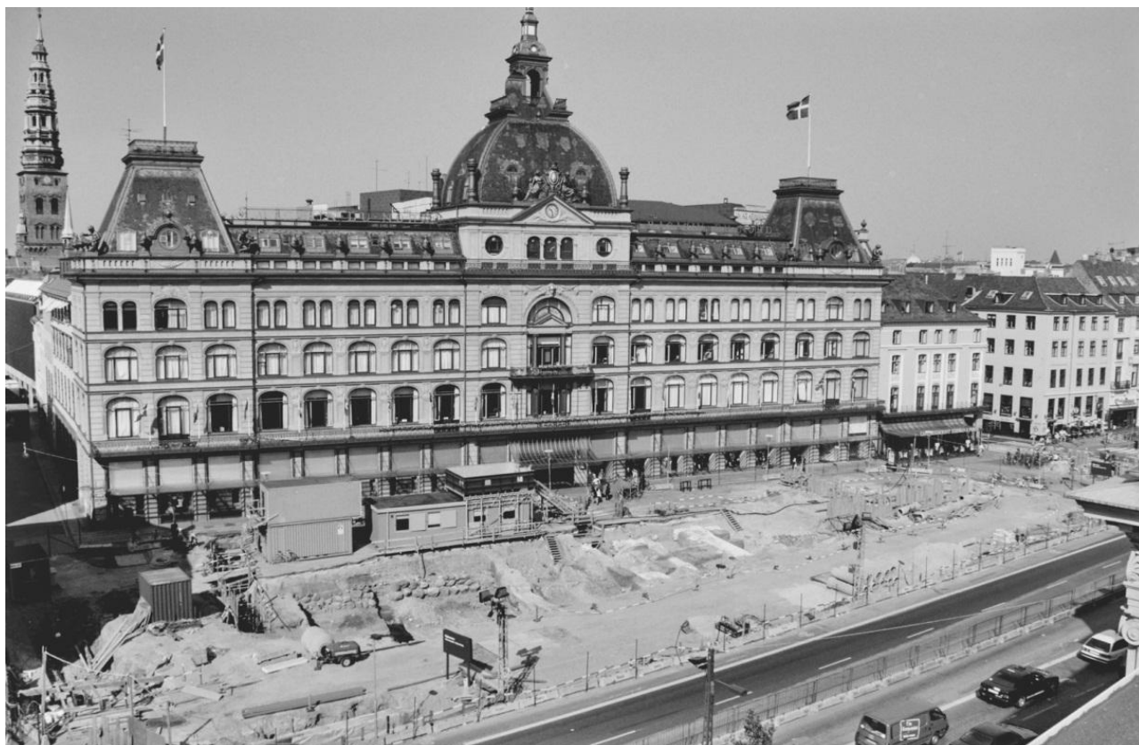
Fig. 9. Overview of Metro excavation in 1996–1998, facing west. Photo: Museum of Copenhagen.
