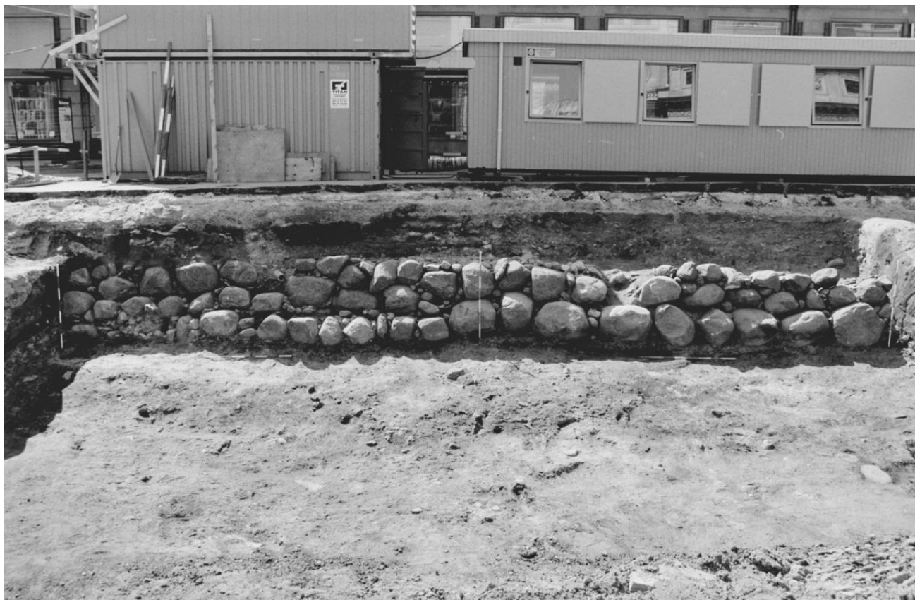
Fig. 12. Interpreted addition to the fortification in the 1580s conducted under Valkendorf's management consisting of a large foundation of boulders, facing west. Photo: Museum of Copenhagen.
