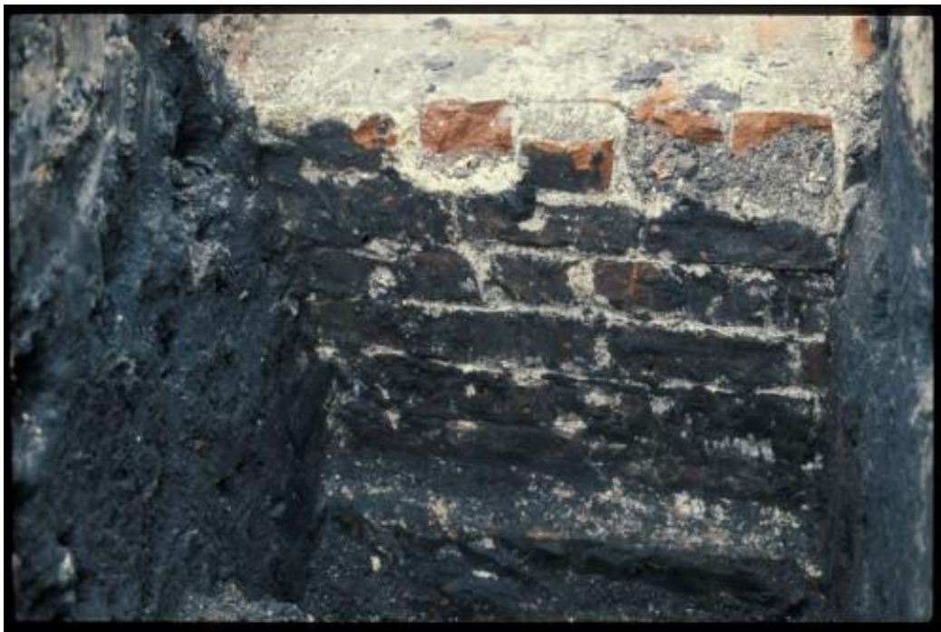
Fig. 15. Part of the brick wall in Vandporten investigated by Bi Skaarup in 1988. Photo: Museum of Copenhagen.
