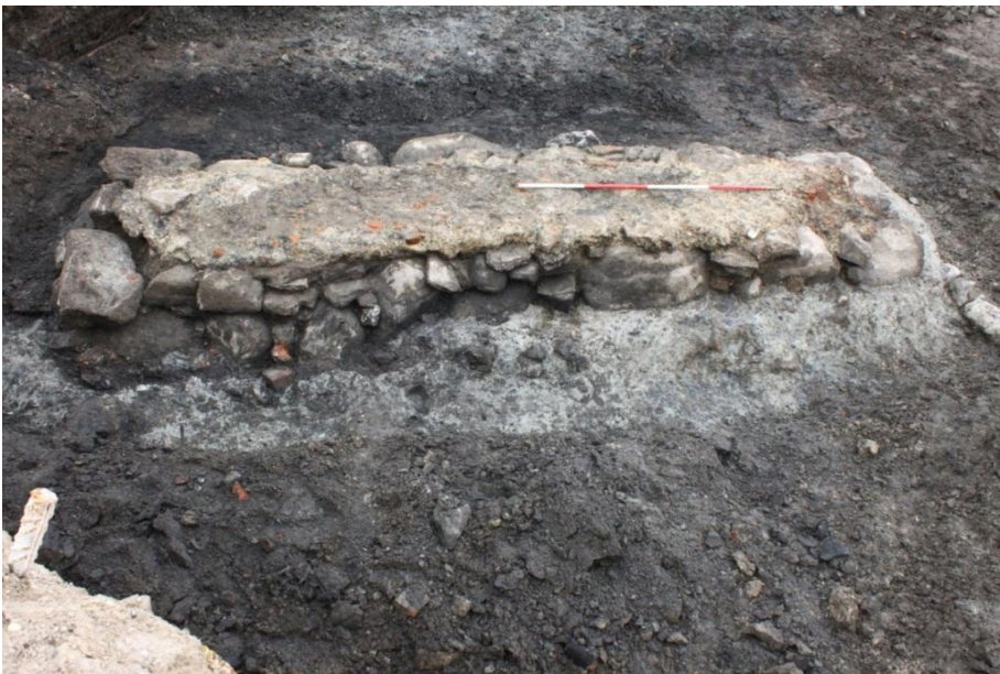
Fig. 180. Bridge pillar No. 4 with foundation and mortar core surrounded by dark waterlogged moat sedimentation, facing west. Photo: Museum of Copenhagen.
