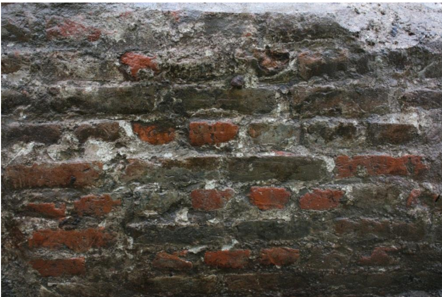
Fig. 187. Close up of brick wall of Dutch or English cross bond, facing NW. This bond has alternating stretcher and header courses, with the headers centred over the midpoint of the stretchers, and perpends in each alternate course aligned. Photo: Museum of Copenhagen.
