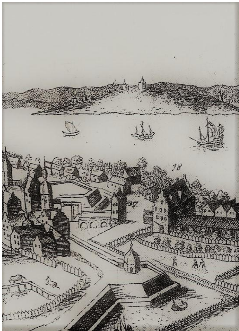
Fig. 198. Part of Johan van Wijck's painting and prospect from 1611 showing Østerport including inner- and outer gate buildings and drawbridge. The Spangenberg's characteristic bastion just north of Østerport is just visible behind the new gate building and is shown as a large, earth-filled plateau with surrounding parapets. A berm is shown by the moat.
