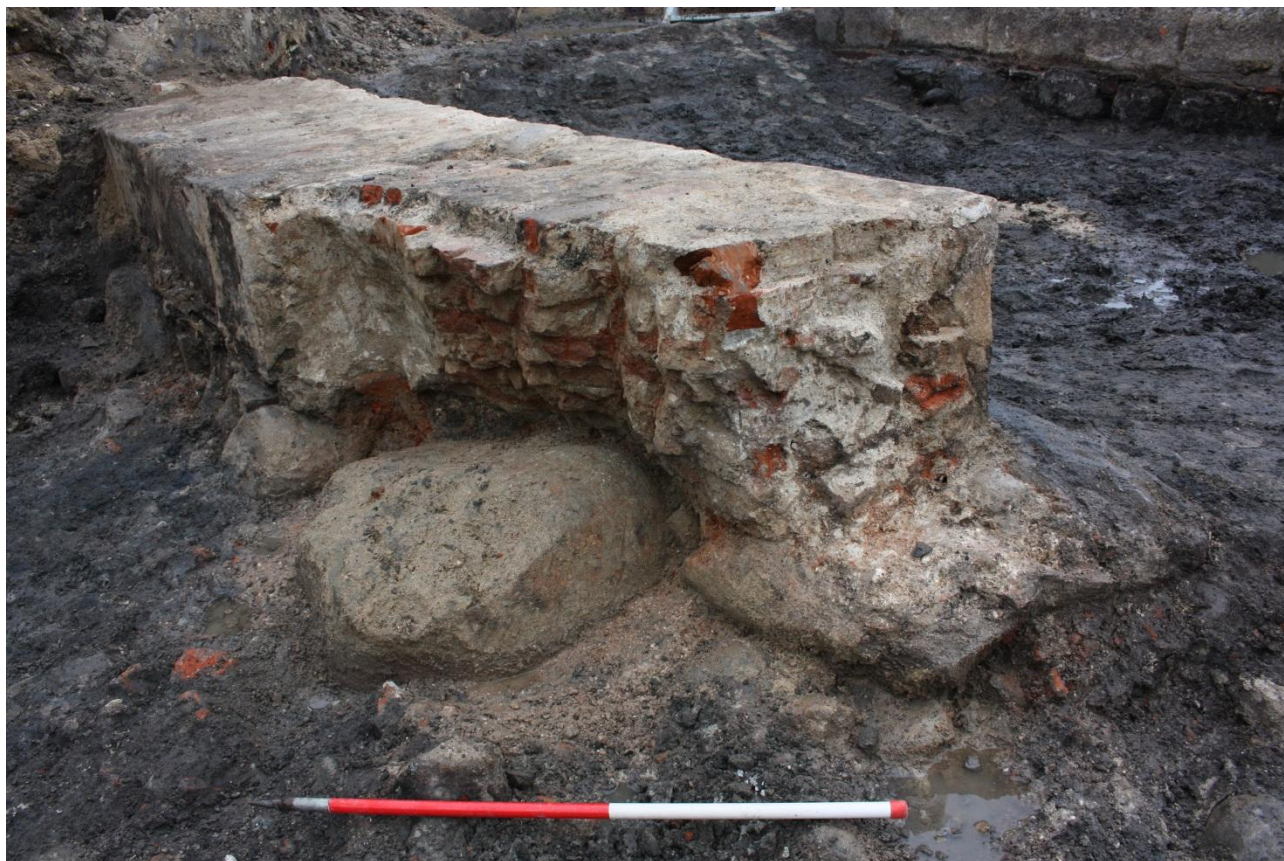
Fig. 176. Exposed bridge pillar No. 1 with foundation, cemented brick and mortar core together with ashlar stones, facing NE. Photo: Museum of Copenhagen.
