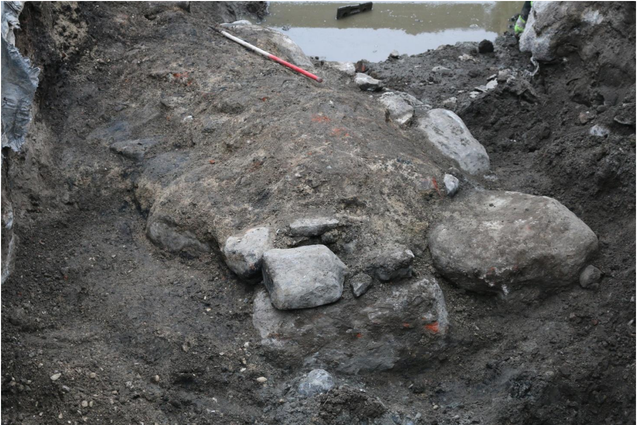
Fig. 181. Bridge pillar No. 5 with foundation stones and mortar/brick core, facing NE. Photo: Museum of Copenhagen.
