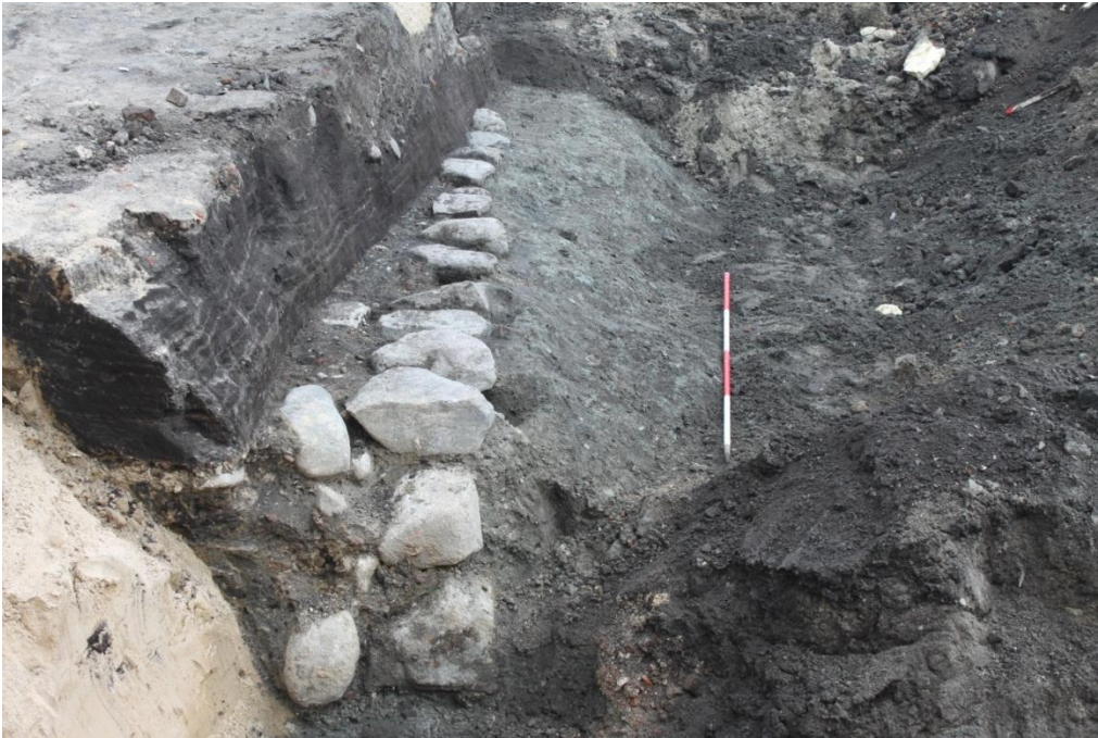
Fig. 156. Southern part of foundation stones in the bastion and sealing clay layer, investigated in 2012, facing NE. Above are multiple layers of peat used as building material in the fortification. Photo: Museum of Copenhagen.
