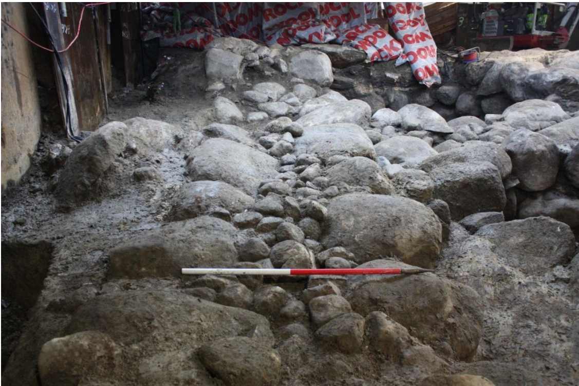
Fig. 79. Construction detail. The southernmost and double faced wall with packing material of smaller stones, facing west. Photo: Museum of Copenhagen.
