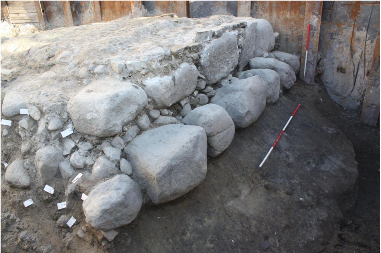
Fig. 63. The eastern face of the city wall foundation with two courses of boulders and intermediate stones and backfills, facing NW. To the right – part of the sloping moat. The structure was truncated by the shoring to the north and the Transformer Station to the south. Photo: Museum of Copenhagen.
