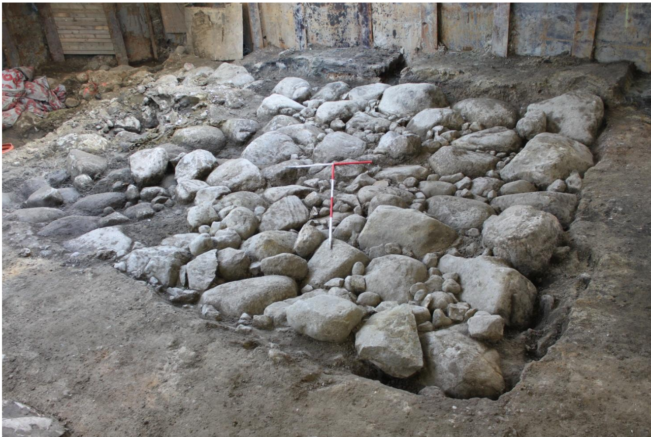
Fig. 77. Southern foundation layer of big boulders and smaller stones dug into natural, facing SE. Photo: Museum of Copenhagen.
