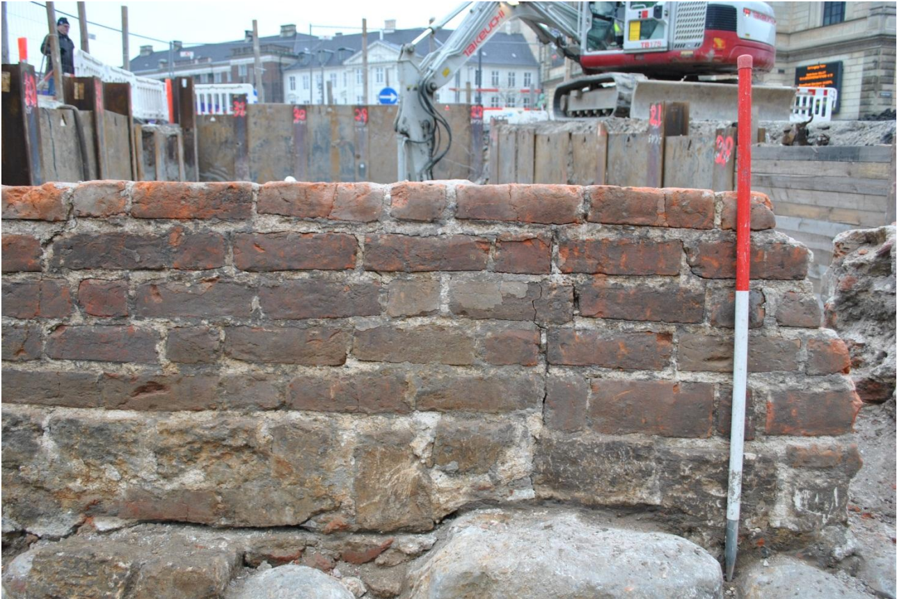
Fig. 68. Detail of brick wall and limestone coursing, facing east. Photo: Museum of Copenhagen.
