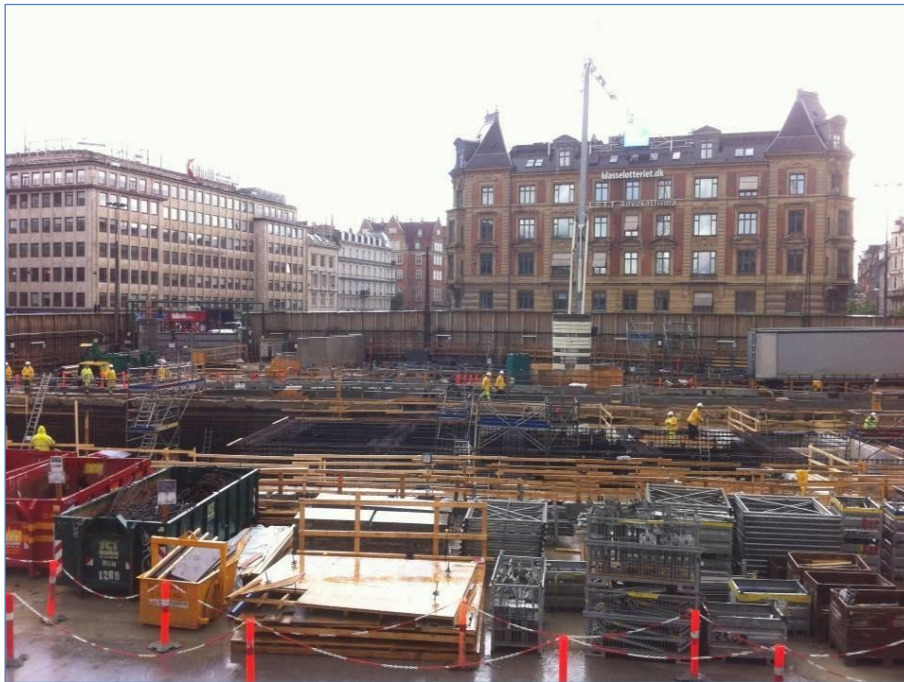
Figure 171 The construction work at Rådhuspladsen, 2013. Seen from southeast
