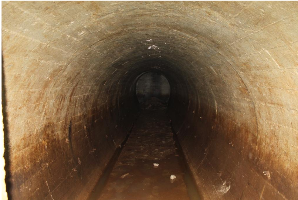
Figure 165 The interior of shelter Group 93
