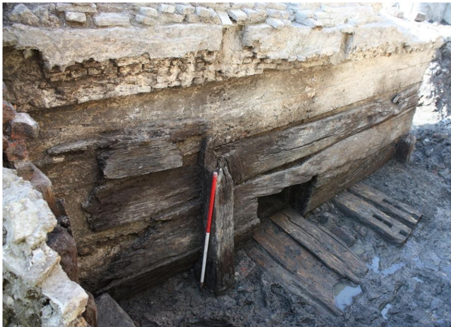
Figure 130 The lowest timber elements southeast of the dam (Subgroups 412 and 356)
