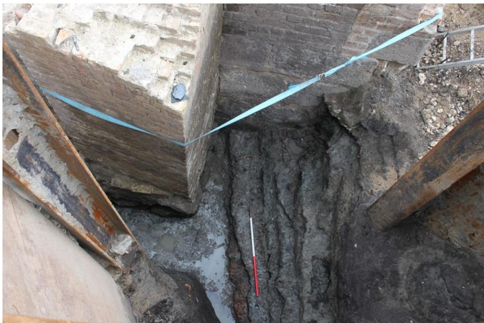
Figure 94 Some landscaping evident in clay placed next to the corner of the outer gate façade
