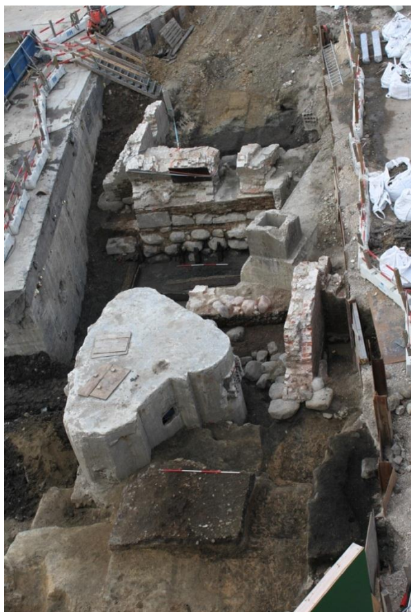
Figure 102 The brick and stone bridge (Subgroup 454) seen from the east
