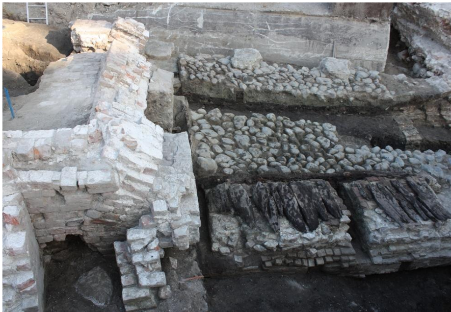
Figure 126b Brick wall, capped in timber, and slot for water (Group 17), all placed within the bridge arch. Seen from southeast
