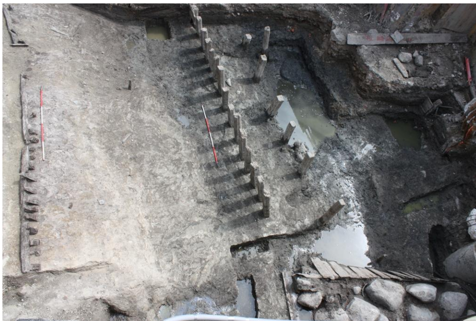
Figure 80 The moat (Group 334) in Area 3 nearing completion, with primary fills still in situ. Seen from above, from northwest
