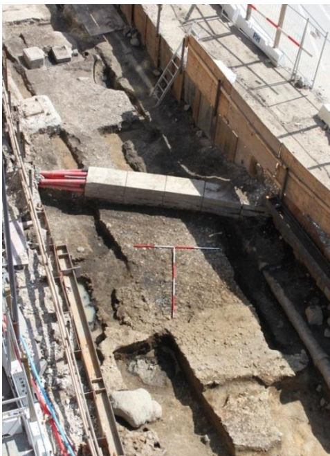
Figure 57 Road surface Group 80 in Area 1, seen from northwest
