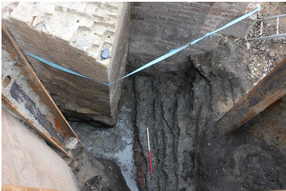
Figure 44 Landscaping evident in clay placed next to the corner of the outer gate façade
