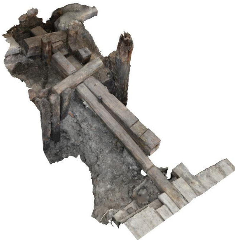
Fig. 120 A photogrammetric rendering of land ties G580 of the Phase 5 harbour and G576 of the Phase 6 harbour, showing how the land ties were related to each other
