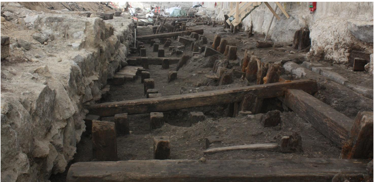
Fig. 145 View of the stone harbour wall looking west shows some of the land ties in situ. In the middle of the picture the anchor beam from G600 can be seen overlying the stretcher beam from G562 from Phase 5, and fastened to it by means of a lap joint and an iron bolt. The square timber posts throughout are the fiskegang from the previous phase, and the truncated anchor beam in the foreground is also from land tie G562 in Phase 5. C03_20140331_9229 (cropped)
