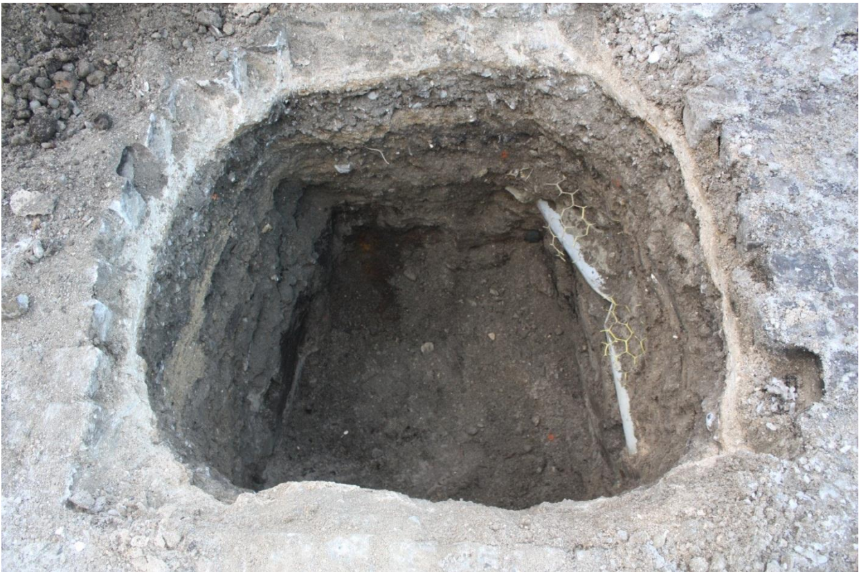
Fig. 374 Working photo of Trench ZT19718 Re-infiltration well. C03_20121220_5536
