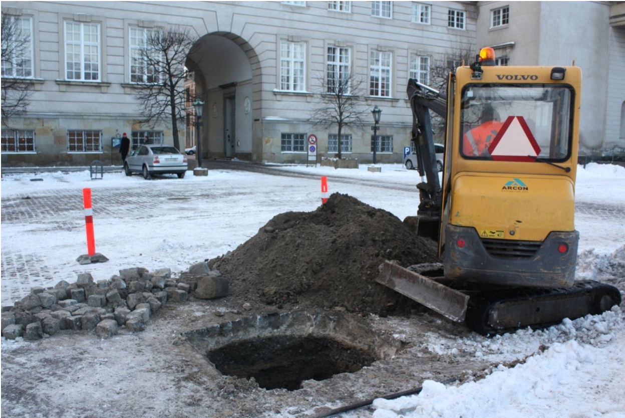
Fig. 373 Working photo of Trench ZT19718 Re-infiltration well. C03_20121220_5535
