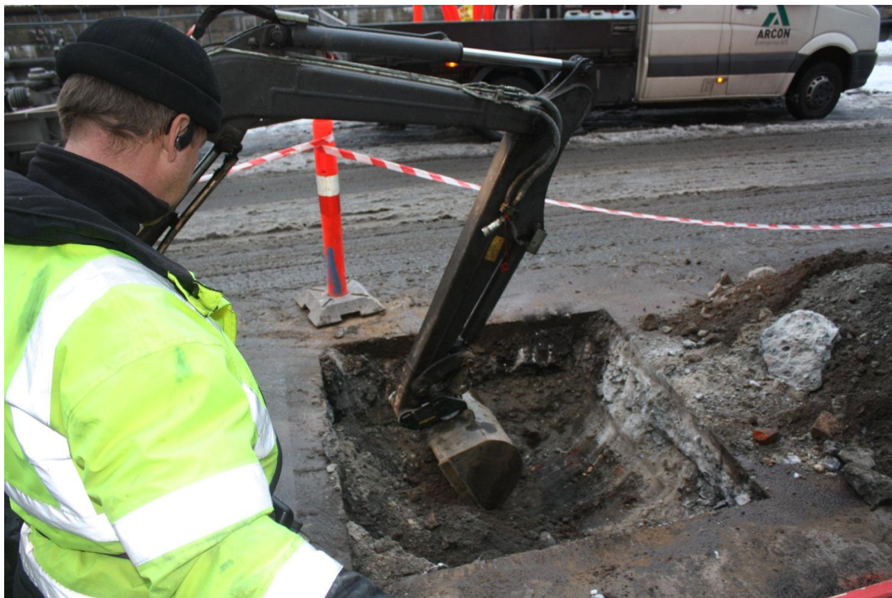
Fig. 372 Working photo of the excavation of Trench ZT19695 Re-infiltration well. C03_20121220_5516.
