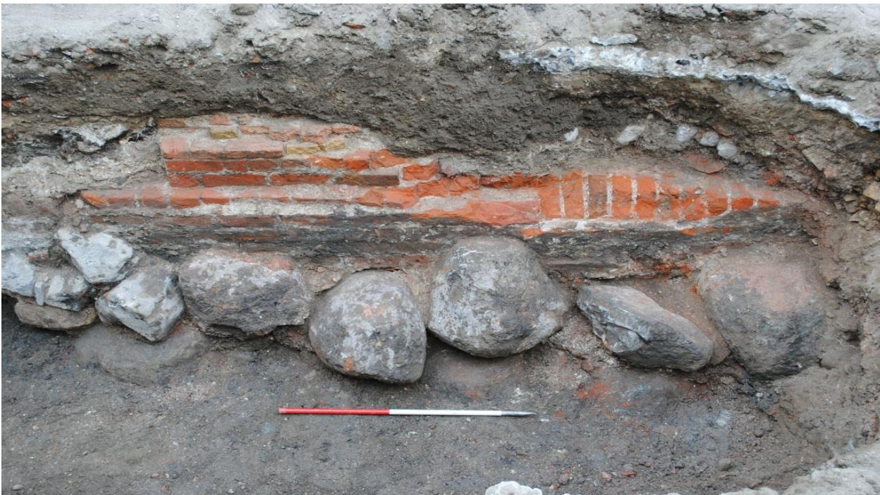
Fig. 49 Northern foundation wall SG220. Comprises Lower course (SS4298), upper course (SS4350) and overlying brick structure (SS4453) C07_20100729_0318
