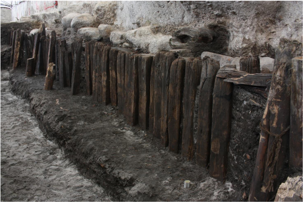
Fig. 46 Photo of central section of harbour wall G532 with bulwark G602 in front. Looking NW.C03_20140611_10788
