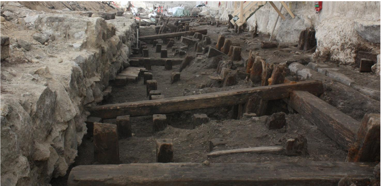
Fig. 350 View of the stone harbour wall looking west shows some of the land ties in-situ. In the middle of the picture the anchor beam from G600 can be seen overlying the stretcher beam from G562 from Phase 5, and fastened to it by means of a lap joint and an iron bolt. The square timber posts throughout are the fiskegang from the previous phase, and the truncated anchor beam in the foreground is also from land tie G562 in Phase 5. C03_20140331_9229 (cropped)
