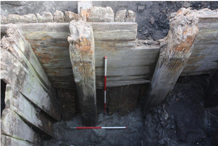
Fig. 327 The excavated planking construction of the bulwark in the Stairway trench. Looking north. C03_20140718_11660
