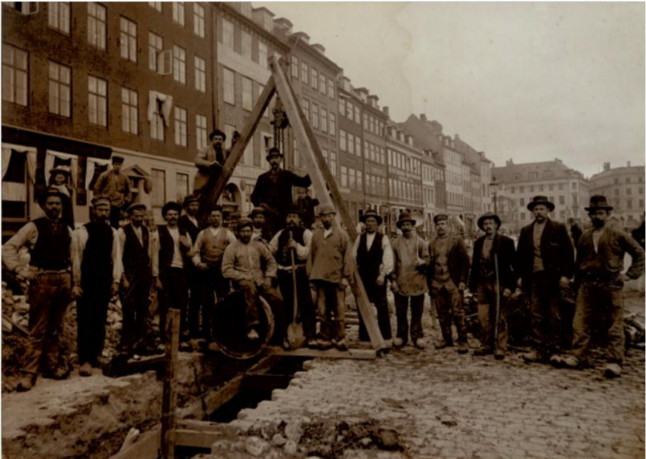
Fig. 362 The large northeast-southwest gas pipe G541 being laid at Gammel Strand during the early 20 th Century. The normal, shorter street lamps can be seen in the background. Museum of Copenhagen
