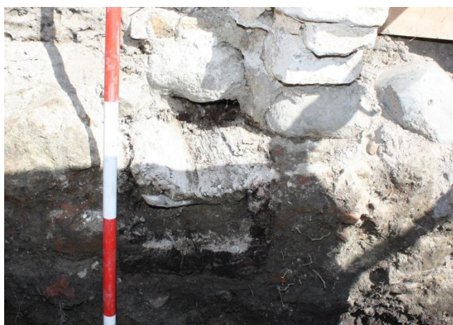
Fig. 284 ST13150 (SG314), partly excavated during the 2012 Guide Wall excavation. Seen in section towards N. C03_20120727_5252 (cropped)
