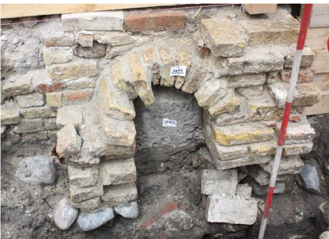
Fig. 286 SS9645 and SD9702, SG423, seen in section in northern edge of Guide Wall trench. C03_280612 4661 (cropped)
