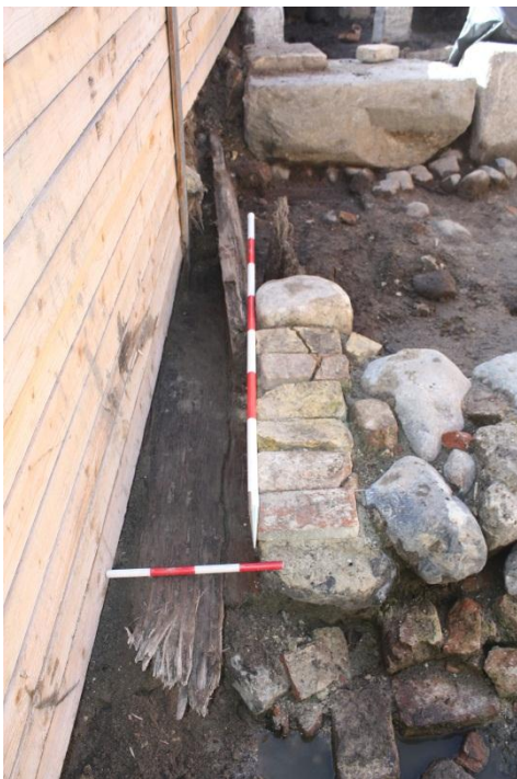
Fig. 280 SS9609 (/SS9127) and ST11222, SG223 excavated during the 2012 Guide Wall excavation. Looking SSE. C03_20120717_4949
