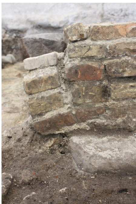
Fig. 252 The short 'stud' wall, SG696, seen here abutting the chimney base SG685 to the right and the robbed out remains of the exterior wall SG693 to the left. Looking NNW. C03_20140311_8681
