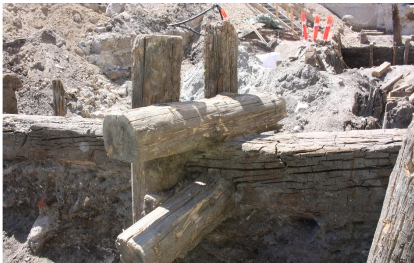
Fig. 151 G653, anchor beam ST47244, with unsurveyed vertical posts and upper and lower rear stretchers, ST53544 and ST39289. Looking SW. C03_20140711_11544
