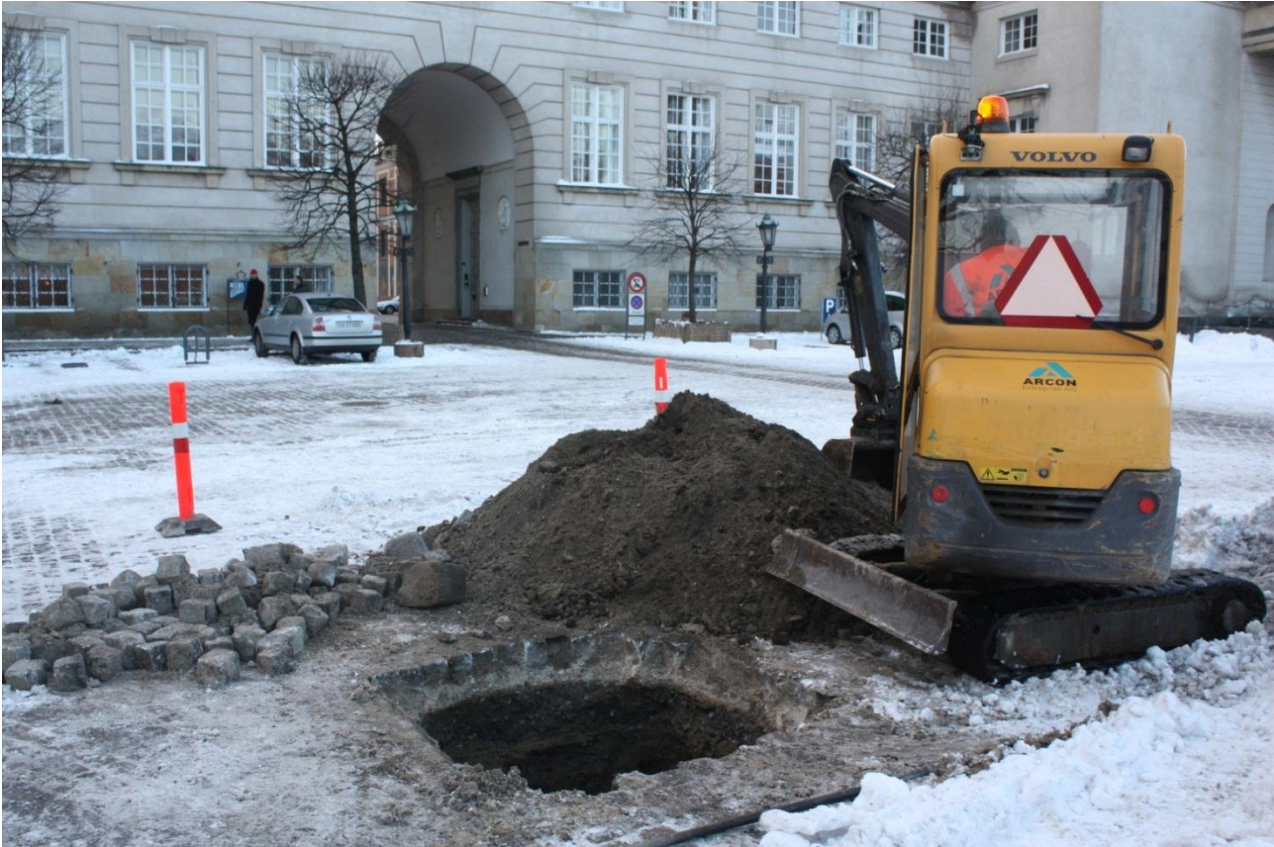
Fig. 8 Working photo of Trench ZT19718 Re-infiltration well. C03_20121220_5535.
