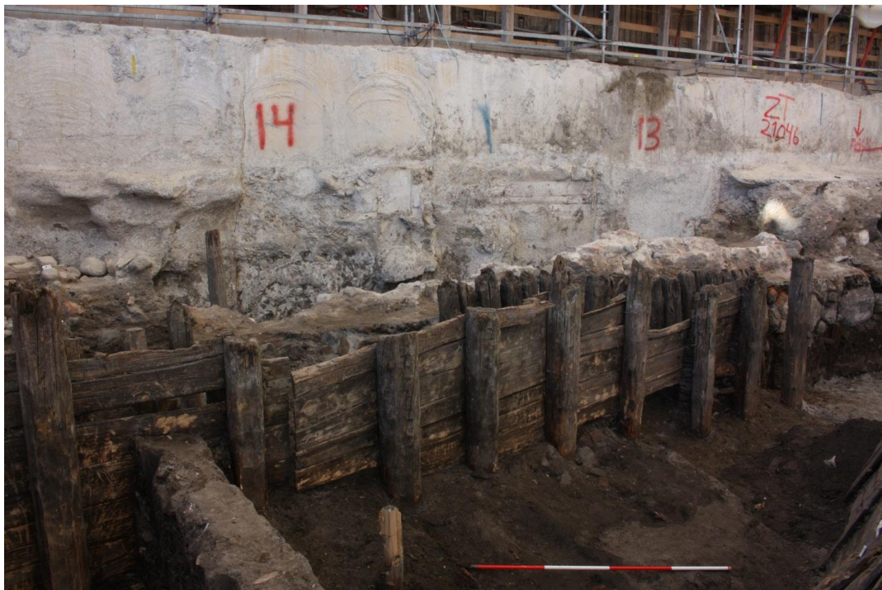
Fig. 87 Reclamation Fence G674, Looking N-W. Note, the bulwark was constructed in two different parts, and that bulwark G602 may have been removed to build this structure. C03_20140624_11187
