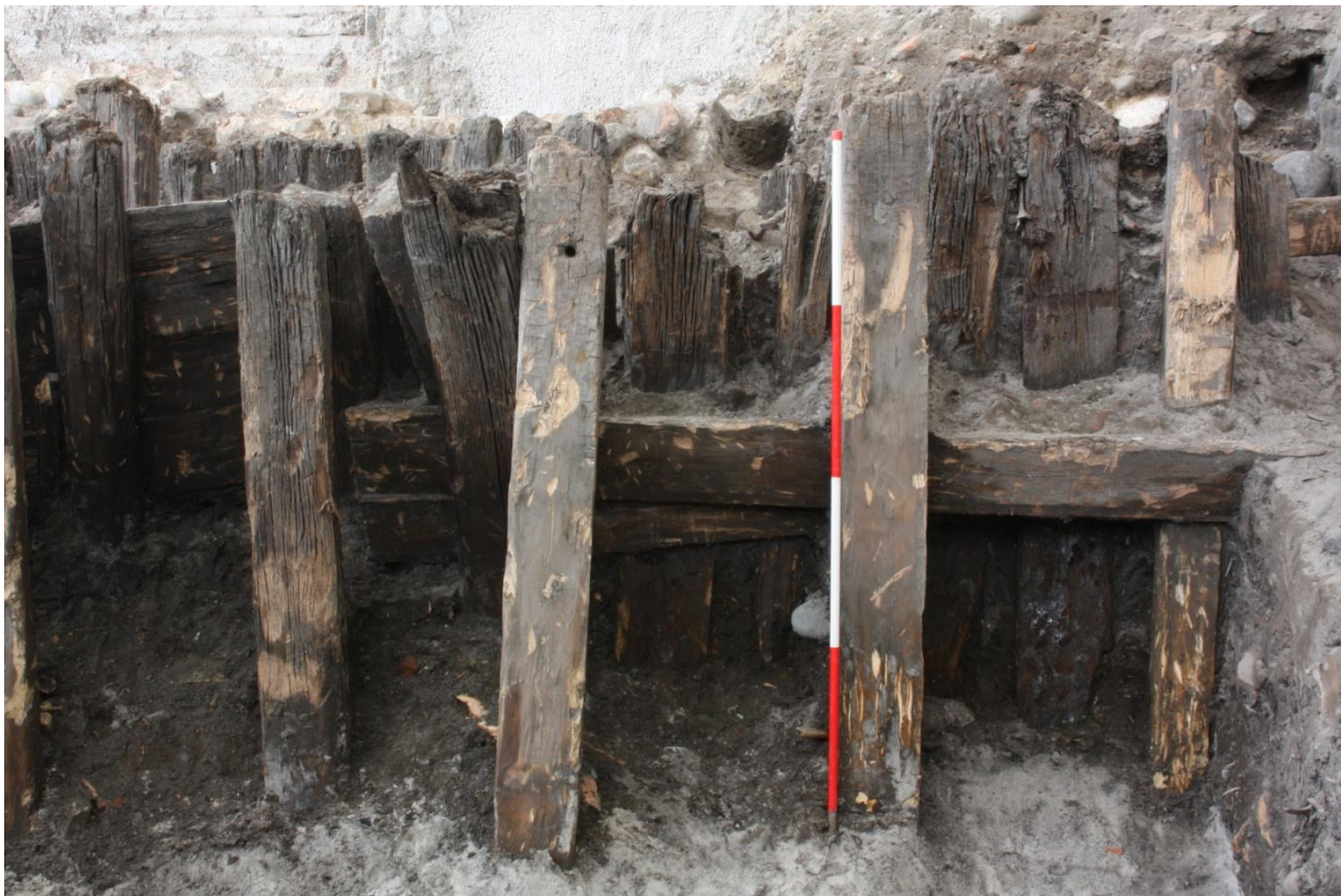
Fig. 94 Close up of harbour bulwark G648 next to the baulk. The photo is centered on an area of repair shown by horizontal plank ST41884 and three vertically set planks (ST39435, ST39413, ST55582) used as the plank's support. The photo is looking N. C03_20140613_10920
