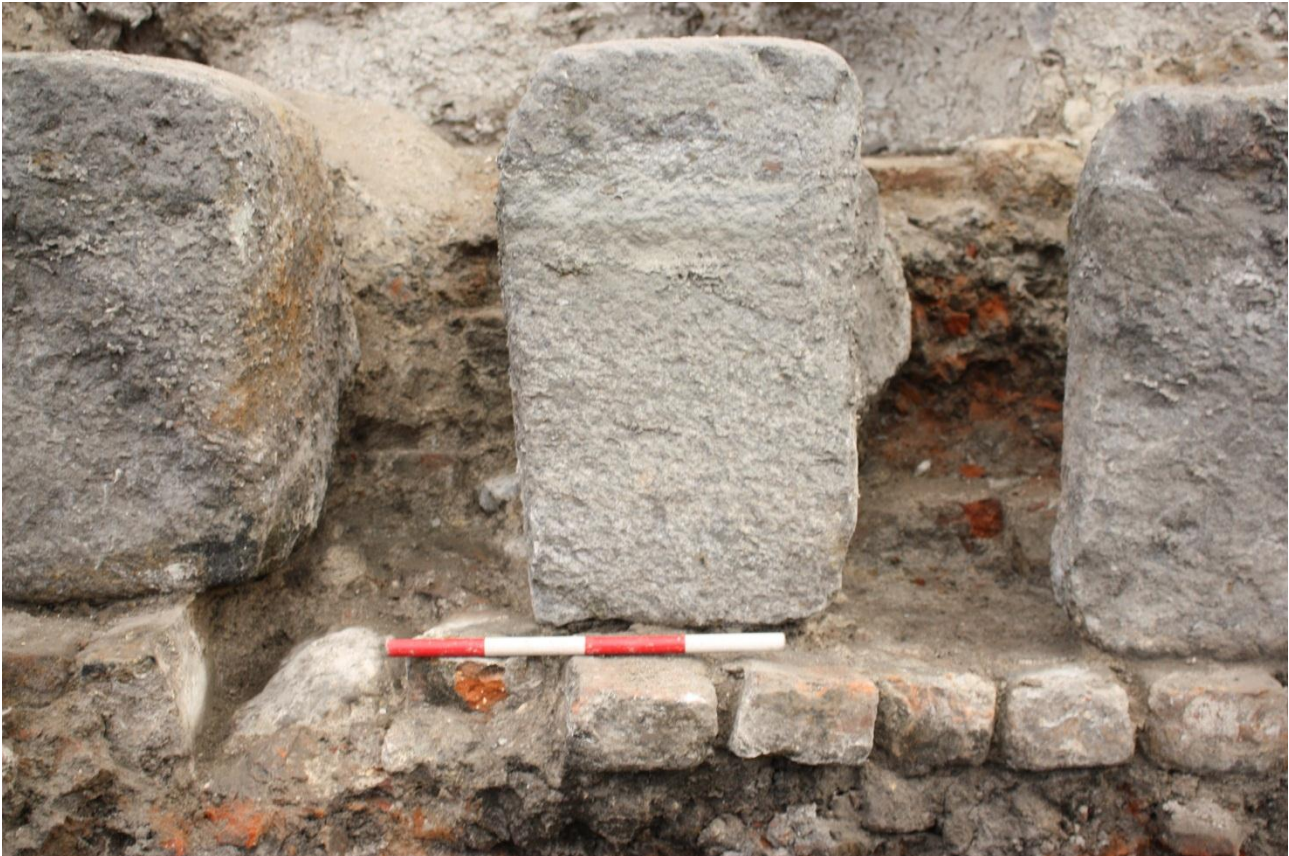
Fig. 73 Photo documentation of the culvert SG477 southern face. Looking north. C03_20140613_10891
