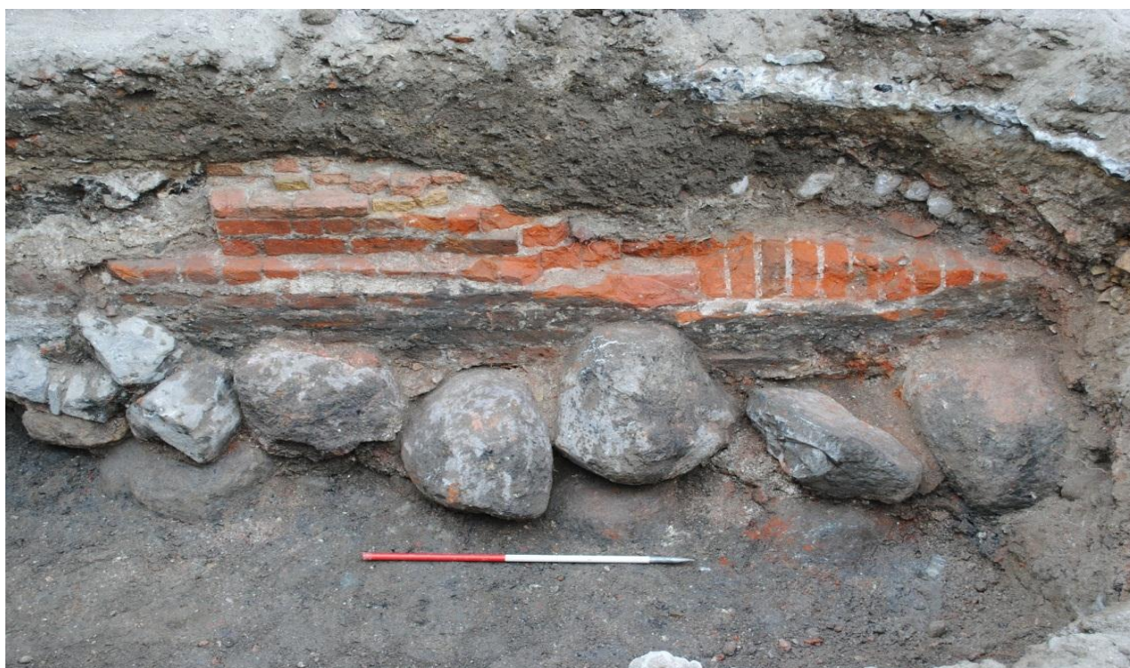
Fig. 60 Northern foundation wall SG220. Comprises lower course (SS4298), upper course (SS4350) and overlying brick structure (SS4453) C07_20100729_0318
