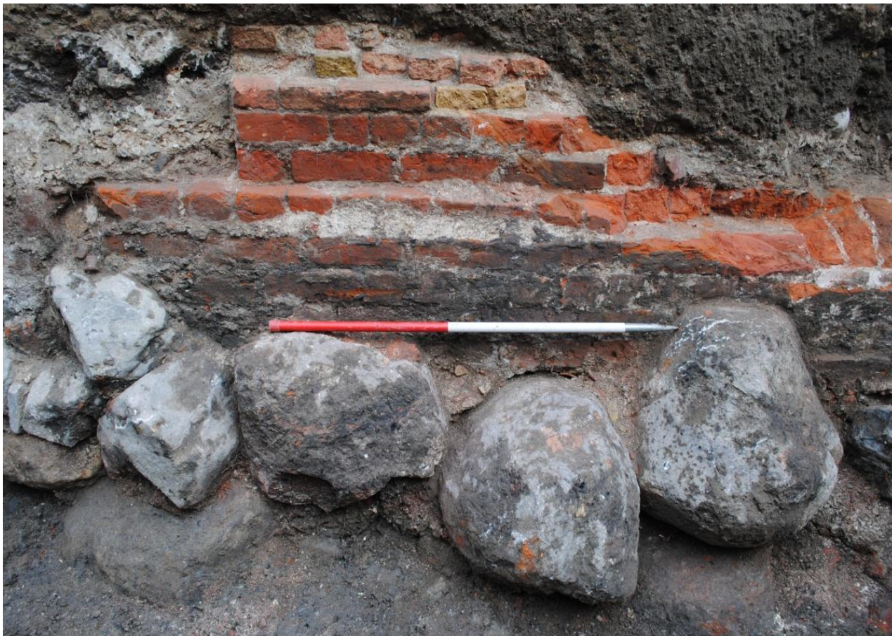
Fig. 64 Northern foundation wall SG220. Indication of a window frame in the upper left corner of the photo. C07_20100729_0322
