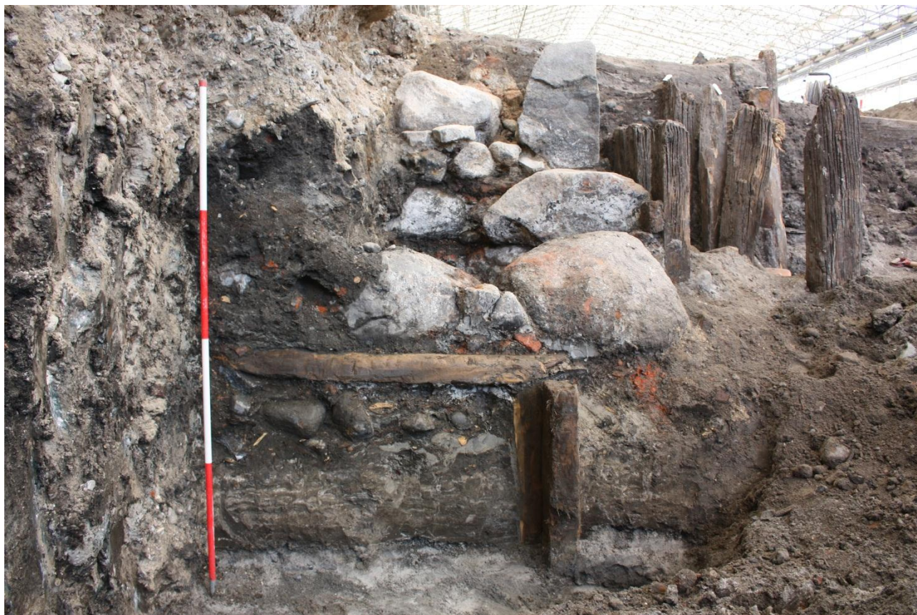
Fig. 70 Photo showing the west facing section of wall G532. Note that the rear of the wall has been truncated, as had the top of the wall by later activity. The Late Medieval harbour bulwark G656 has been cut or snapped with the upper part of the post horizontally placed on a north-south orientation C03_20140630_11307.
