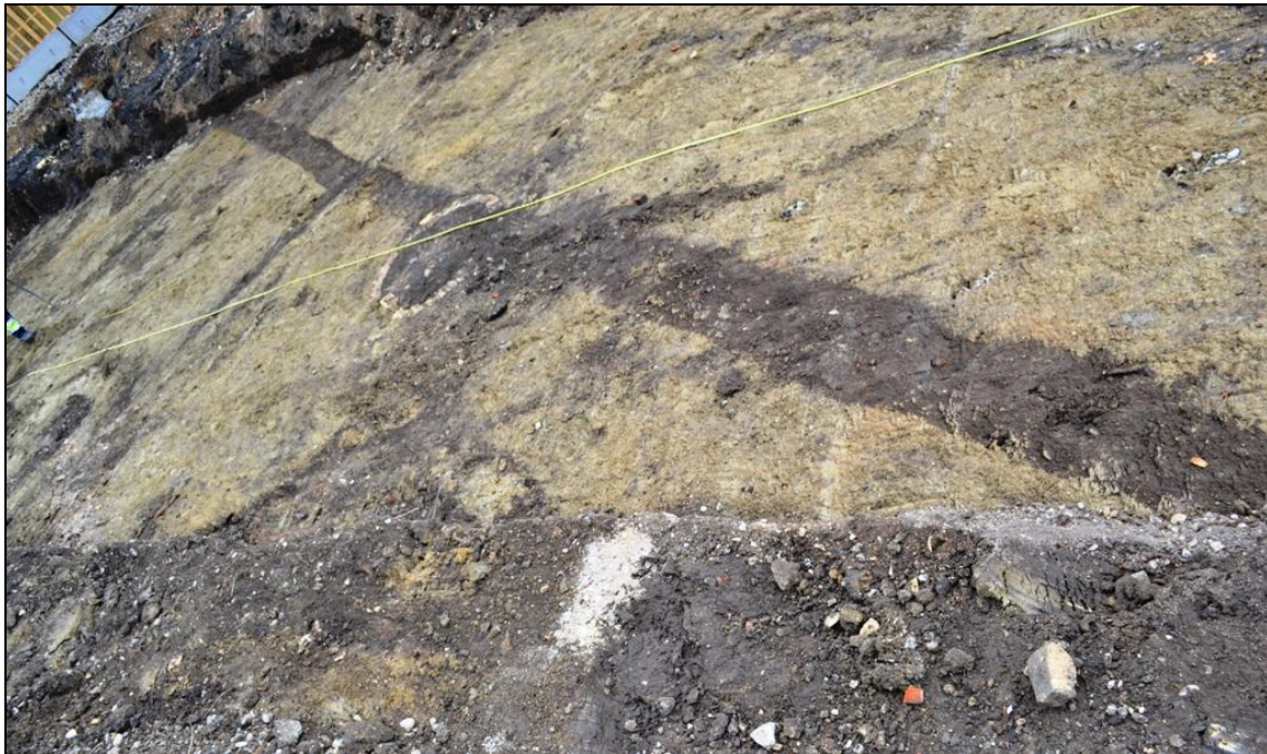
Figure 19. Drainage ditches and brick well S100005 in the south end of the construction site.
