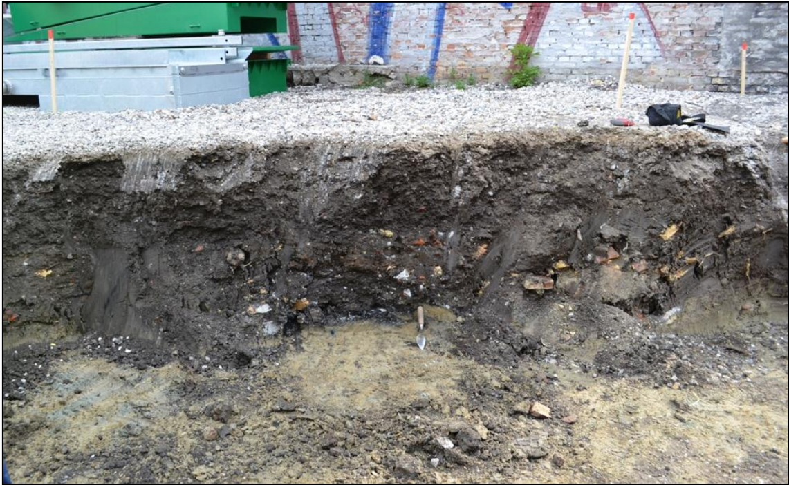
Figure 16. Overburden above the natural subsoil containing fragments of bricks and tiles.
