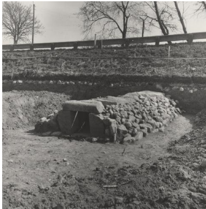
Figure 13. Culvert from the 1800s excavated at Hasselager in 1985 by Moesgaard Museum. Photo: Forhistorisk Museum Moesgård.
