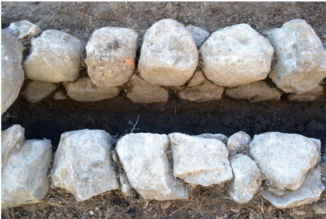
Figure 12. The upper course of stones is resting on a lower course that has been laid in a trench dug into the natural subsoil.
