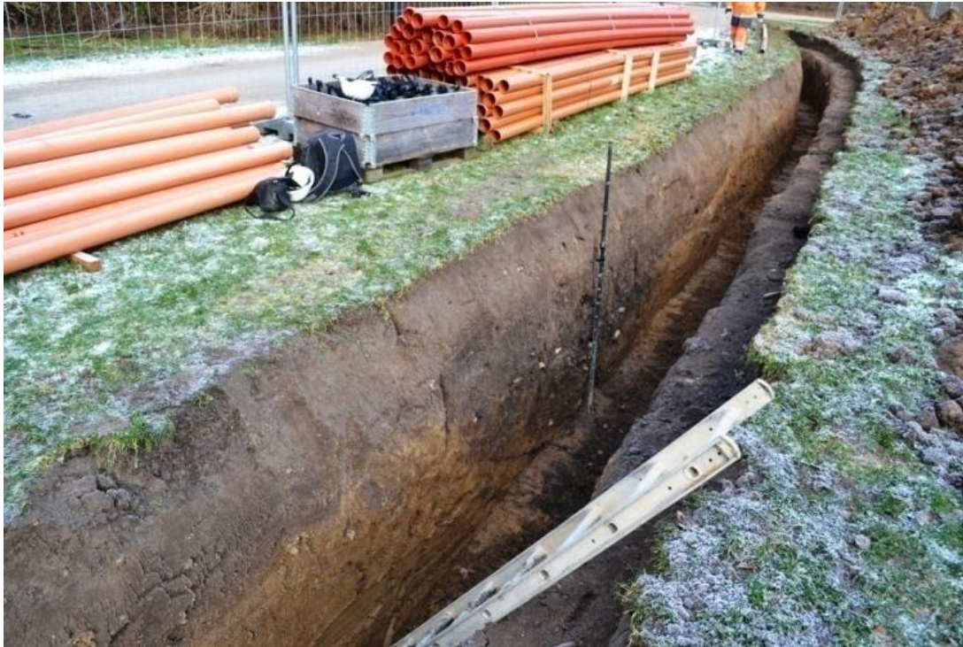
Figure 8. Trench 1001 with Pit S1033.
