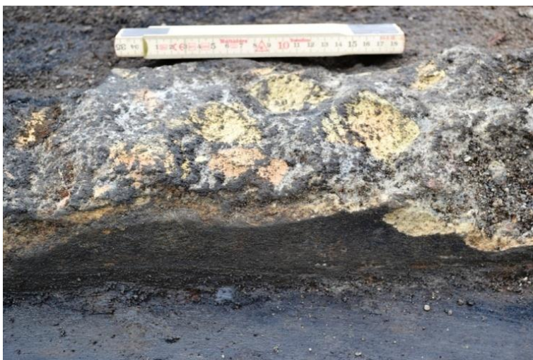
Figure 14. A layer of mortar covered the floor and extended up the crushed-brick mortared walls (S1008).
