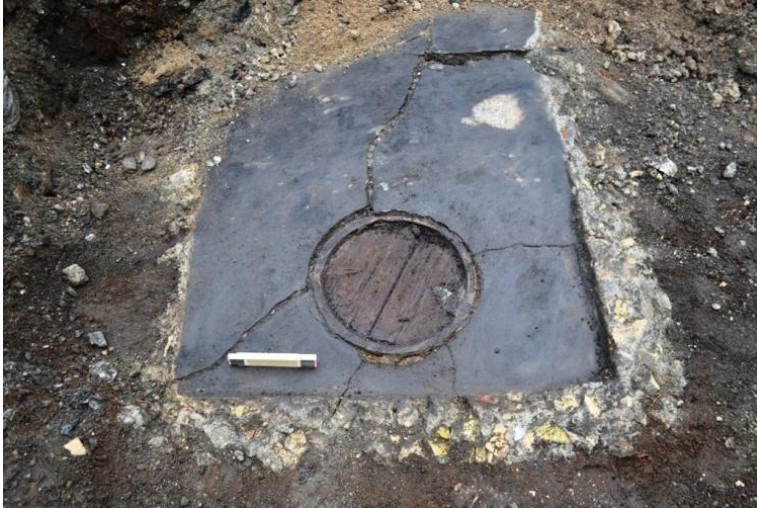
Figure 12. Floor drain in the car garage covered by wooden lid (S1008).
