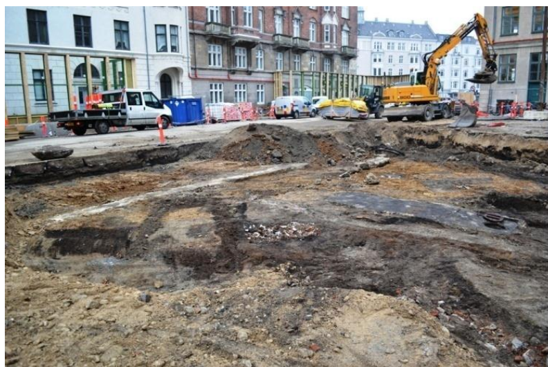
Figure 11. Foundation wall S1056, the mortared floor S1008 and an accumulation of ceramics and other household debris (S1012).
