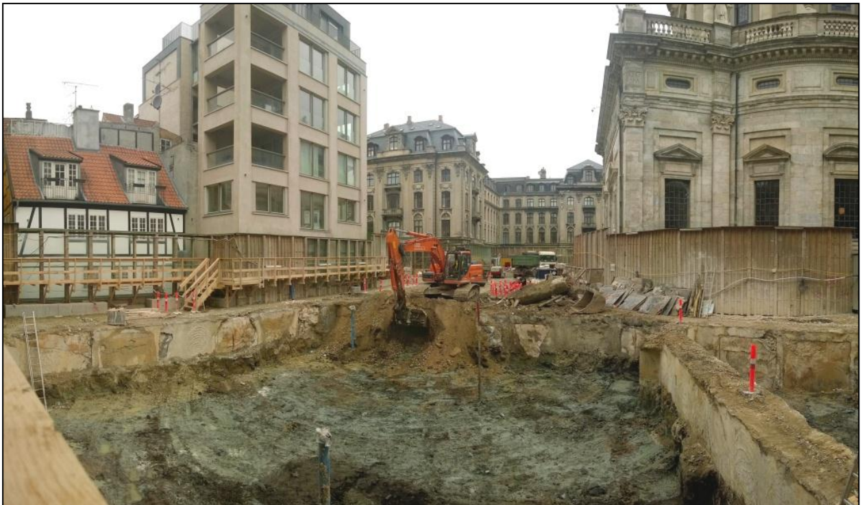
Figure 12. Excavation of the station box southwest of the church in 2014.
